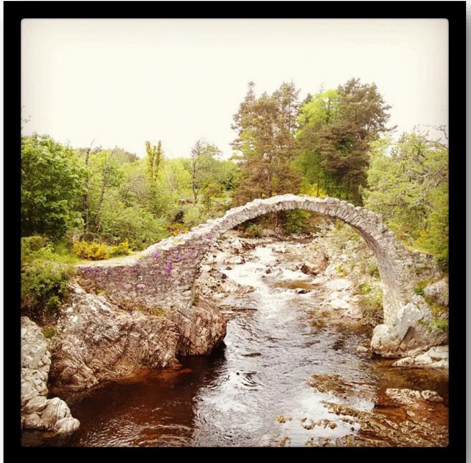
A really old bridge at Carrbridge #1e109947
